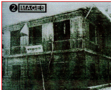
The old Facoma building that housed the fledgeling school.
